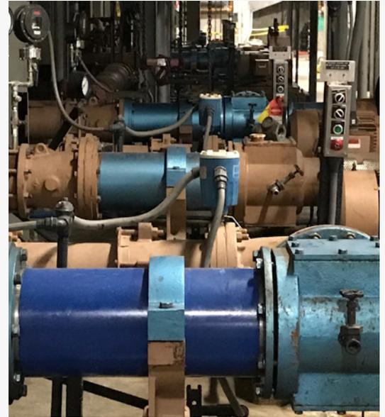
The Moyno 2000 2K800G1 offers the maximum combination of pressure and flow rate in comparison to any progressive cavity pump made. Installed in 1994, the pumps continue to deliver value by operating with minimal maintenance.
