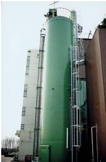
Installation for lime metering in a waste water treatment plant
