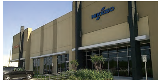
We stock pumps at our Houston, Texas office for quick delivery.
